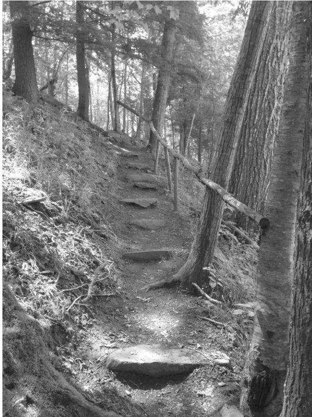
Steps under repair in August along the Great Pond Trail.
