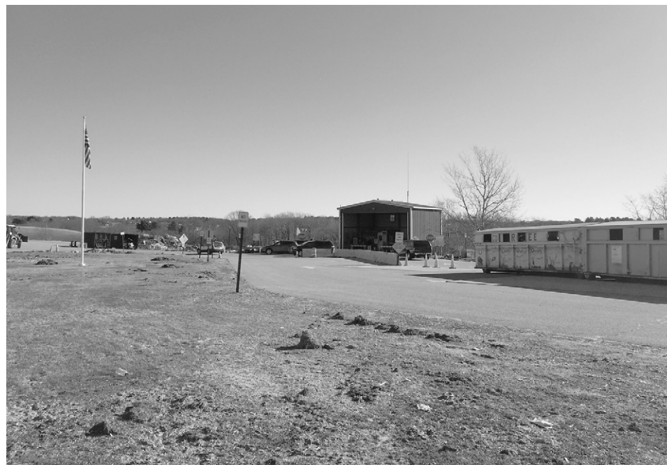
In June, voters will decide whether to approve a $1.4 million bond to finance improvements at the Recycling Center. Above, the Recycling Center as seen on Saturday morning, Feb. 27.
