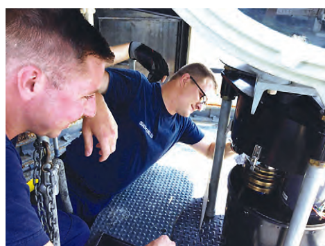
U.S. Coast Guard Electrician Mate 1st Class Tony Robb and Electrician Mate 3rd Class Alex Trade repairing light.
