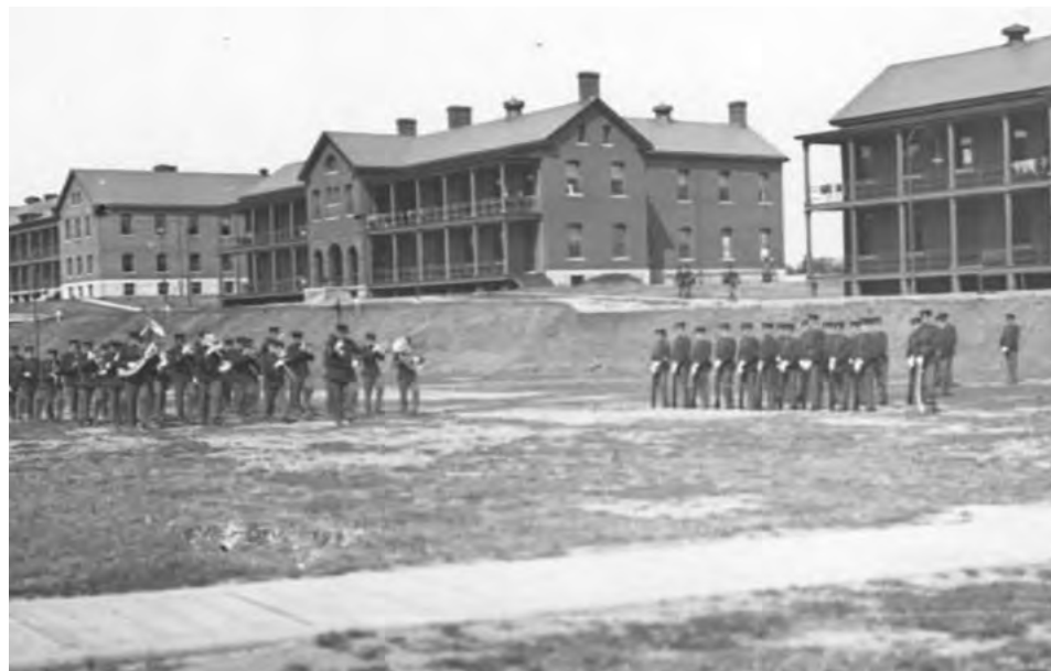
Photo courtesy of CEHPS
